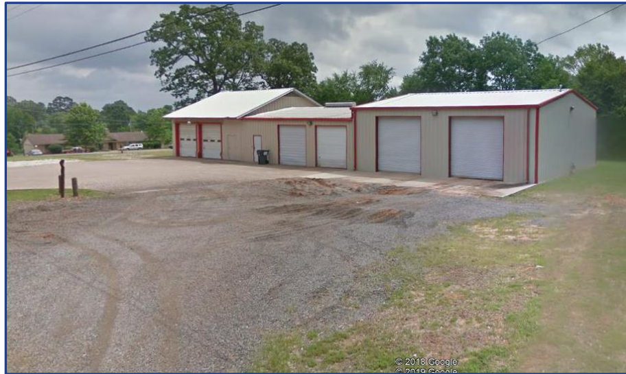
Figure 5: Jackson Heights Station 1 Driveway and Apparatus Pad
